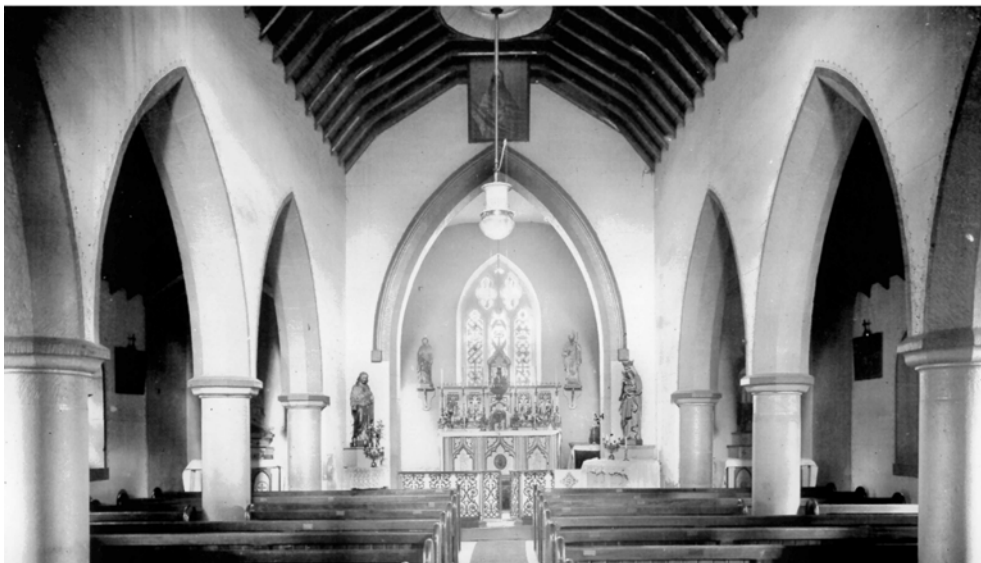
The interior looking east, c.1912 (Mitchell Library, State Library of New South Wales, Hazlewood Collection, ON165/147)
